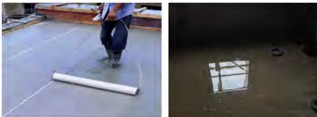
图 50 覆盖薄膜和蓄水养护
